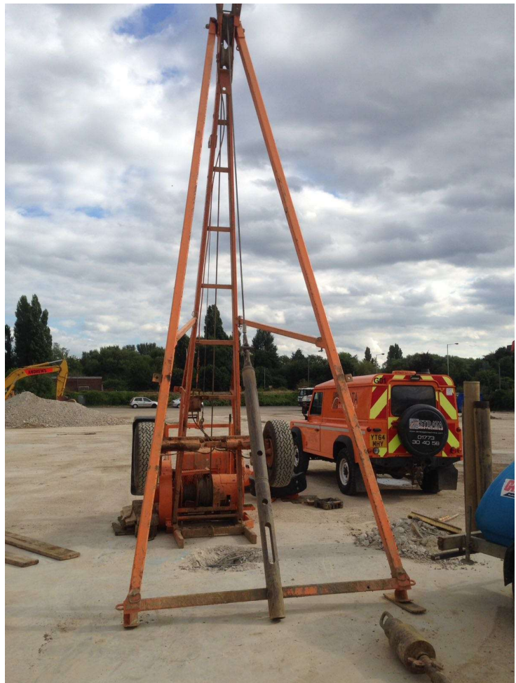
Figure 1: Cable Percussive Rig set up and ready for operation
